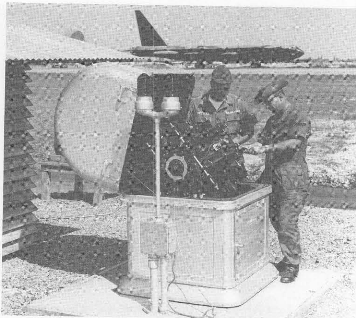
Adjusting AN/GMQ-13 rotating beam ceilometer at U-Tapao Royal Thai Naval Air Station (RTNAS), Thailand, in 1969 are Sgts Raymond J. Metzge (left) and Robert W. Stalker from Det 30 of 1WG's (1WW) 10WS. In background is SAC B-52 on landing roll.
