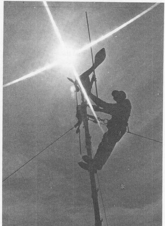
Weather equipment repairmen in AWS—the end of an era.
